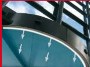
**Air curtains.** Minor drafts can be excluded by a warm air curtain. The heat can be provided by the building's heating system.
